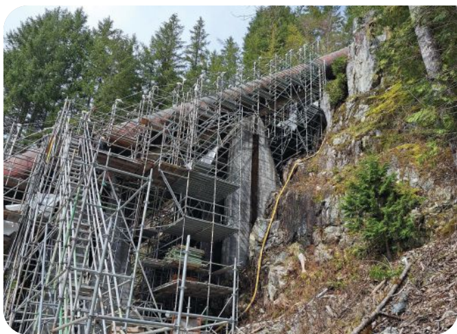
Scaffolding was constructed around the BC Hydro penstocks prior to exterior surface preparation, which included abrasive blasting operations.
