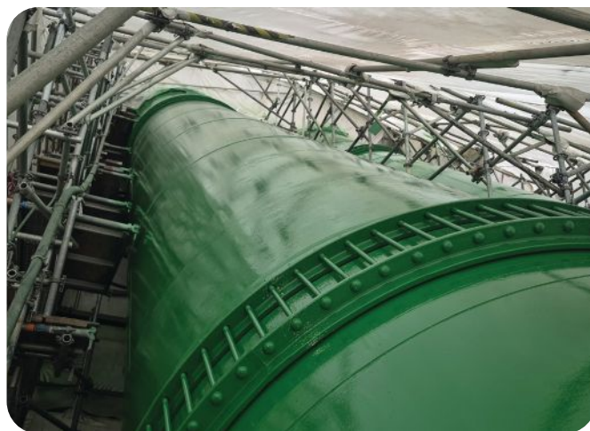
The penstocks’ exterior surfaces received one coat each of Carboline’s Carbozinc 859 zinc epoxy primer, Carboguard 635 HAR epoxy, and Carbothane 134 HG at approximately 10–20 mils.
